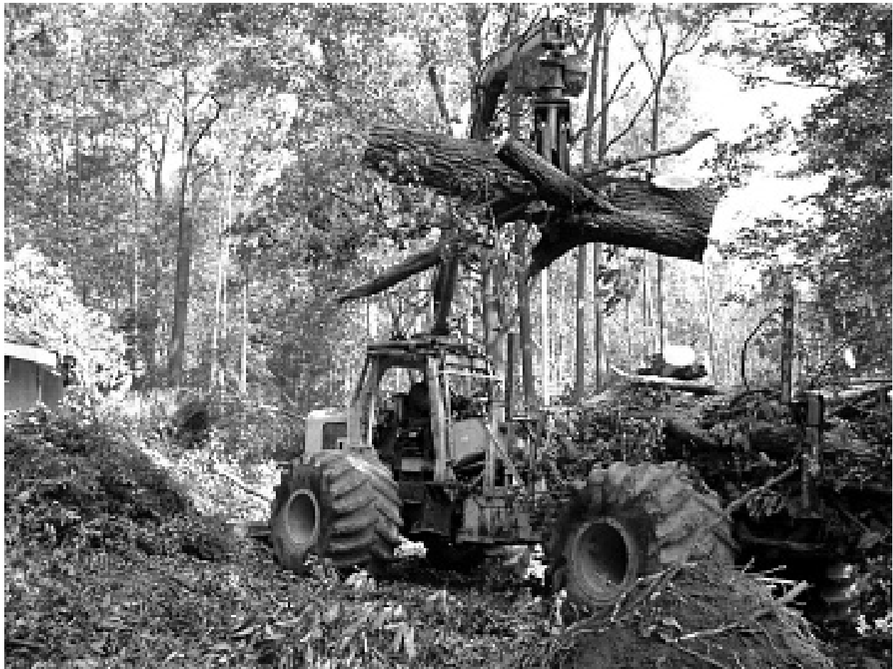
Tree being lifted by heavy equipment in the Sauer's garden. Note the house at left edge of photo. Photo by David Sauer.
