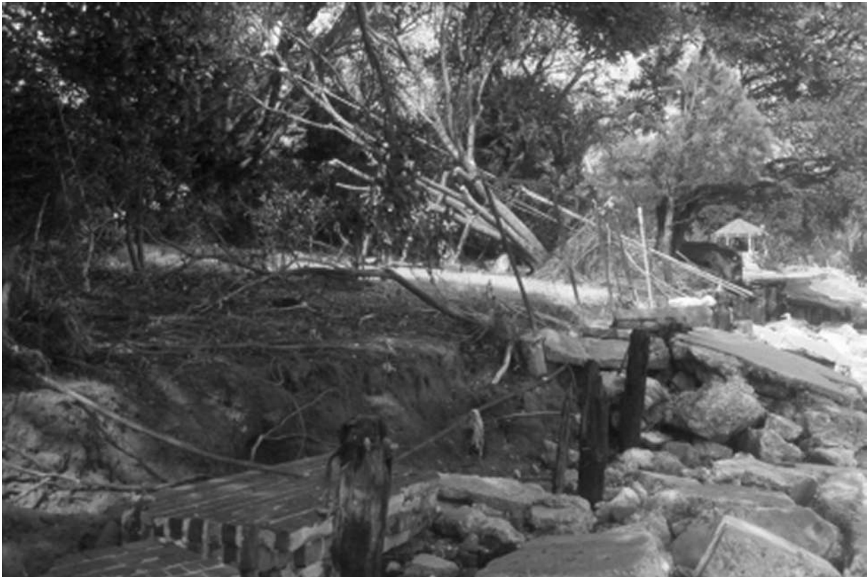
McDonald's demolished seawall, brick wall, fence, and vegetation in Hampton. Photo by Ken McDonald.
